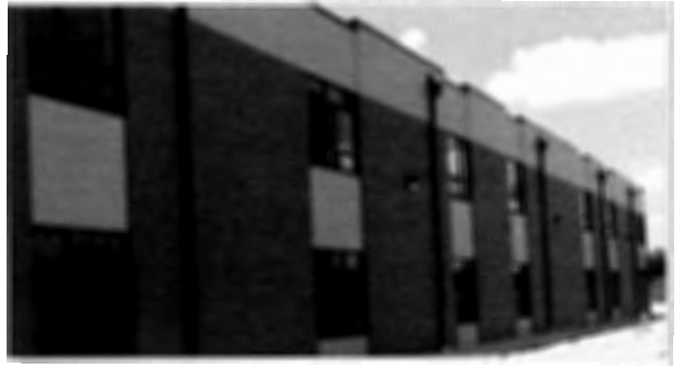
New Linn Elementary School – Classroom Wing
